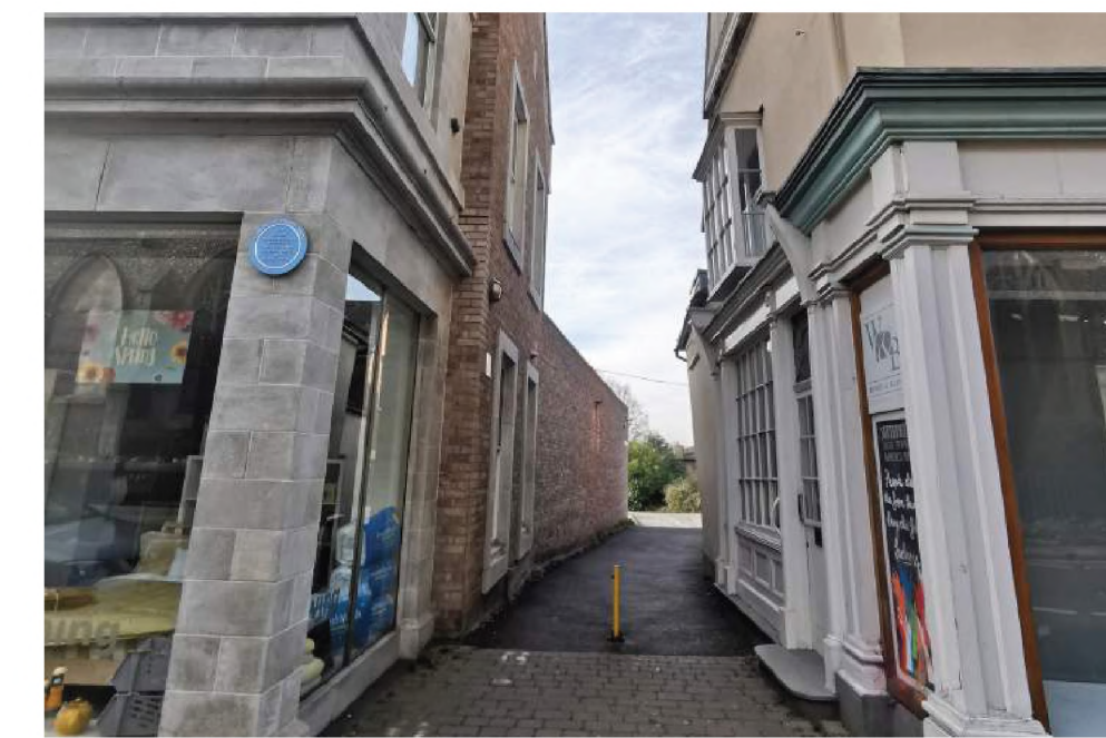
Existing block penetration
