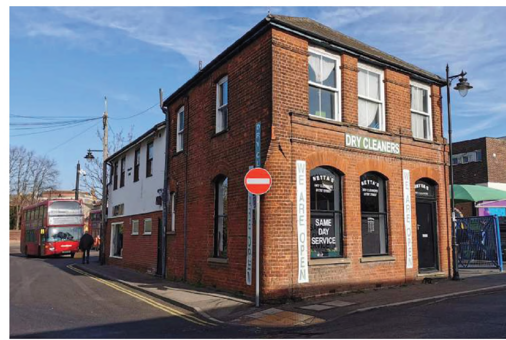
Locally listed – “should be preserved as a good example of a late Victorian commercial office”
